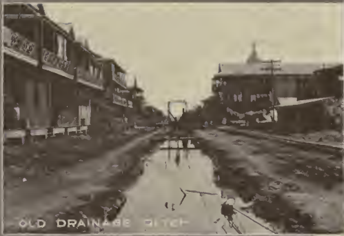
OLD DRAINAGE DITCH
